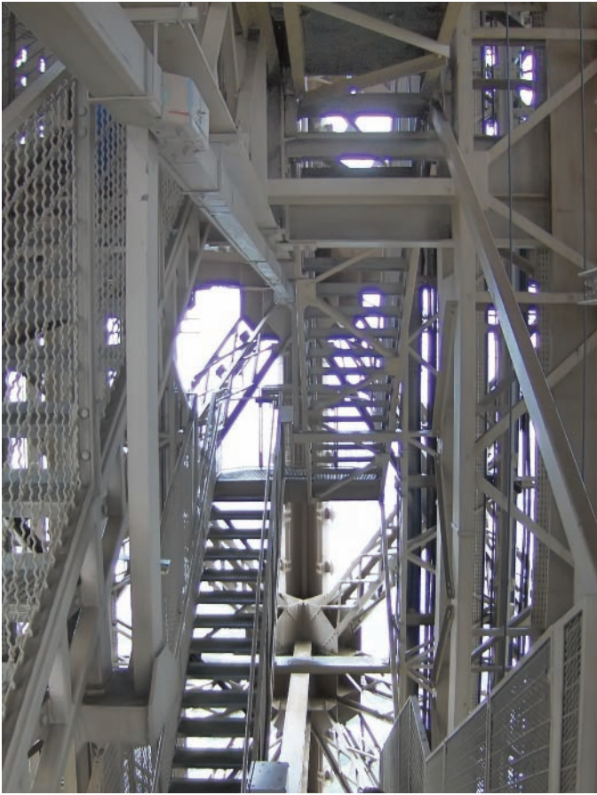
Fig. 9. Service stairwell underneath the summit. Credit: France Languérand.
