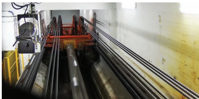
Fig. 5. Chariot pulling the cables in the subbasement. Credit: France Languérand.
